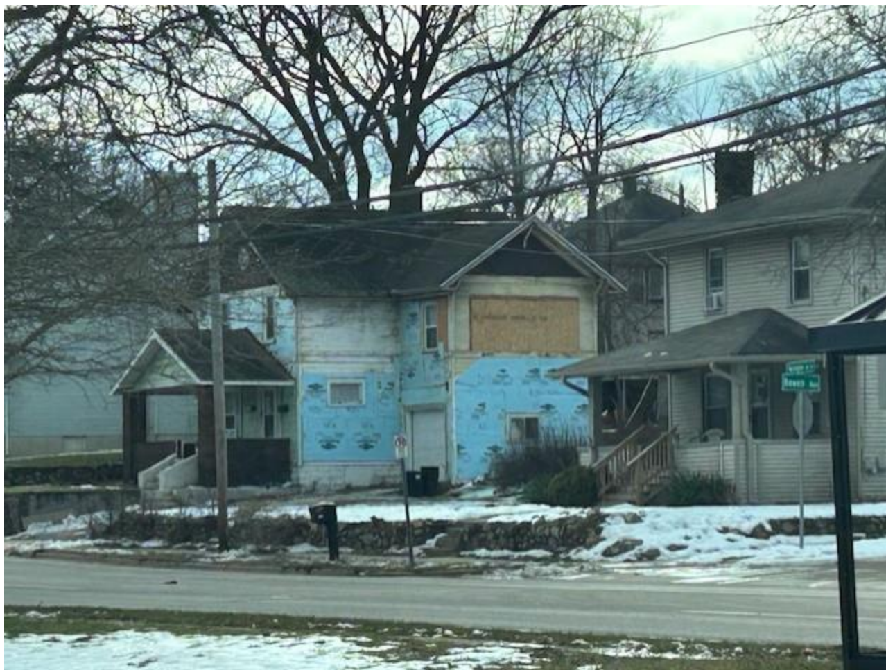
Figure 3: Street view of the subject structure at 263 N Washington Ave., taken February 4, 2025. Much of the existing siding had been removed from the structure, exposing the previously covered cedar shake siding near the peak of the home.
