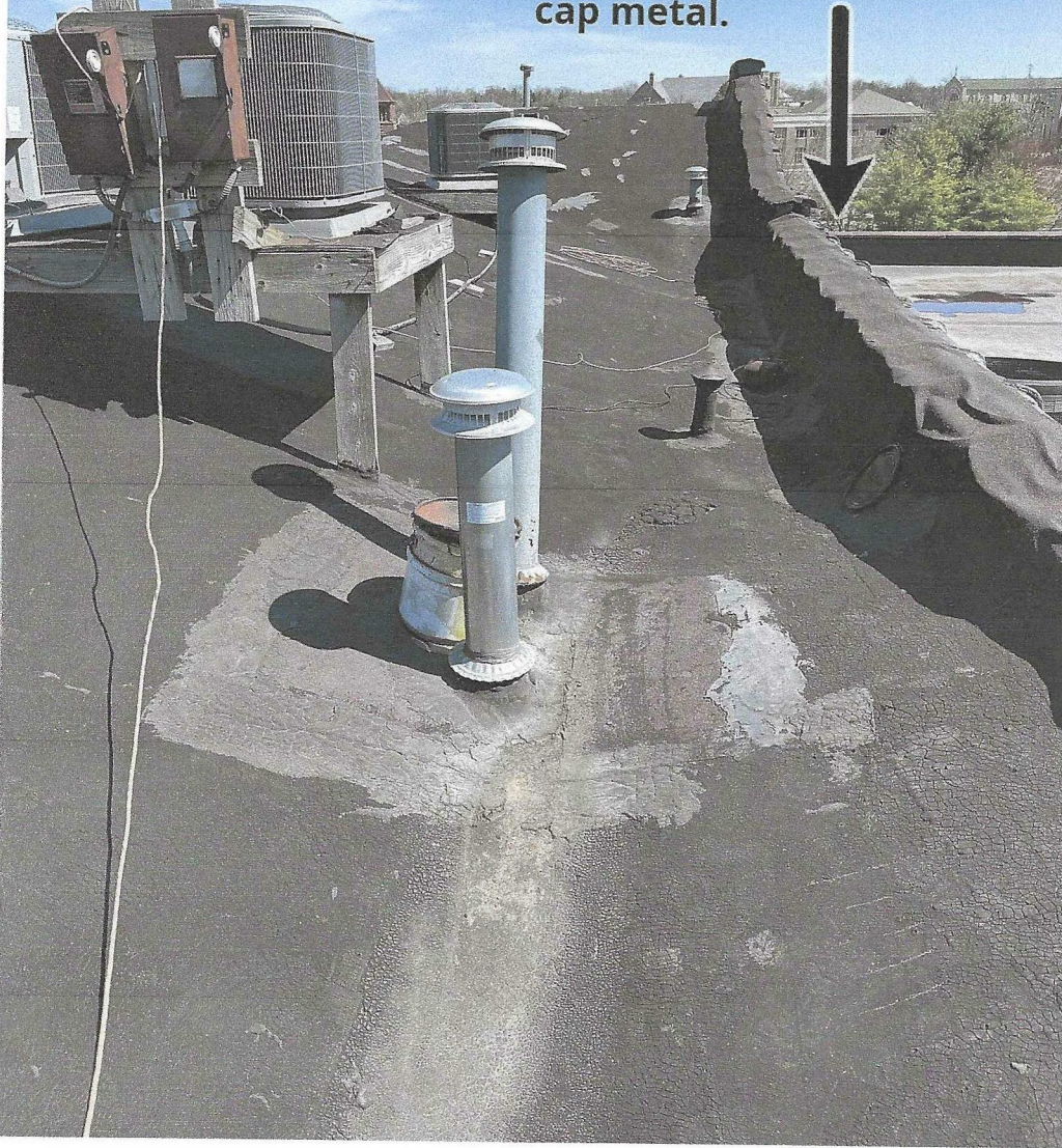
Photo Description: Metal cap is 2 pc compression drip style.
