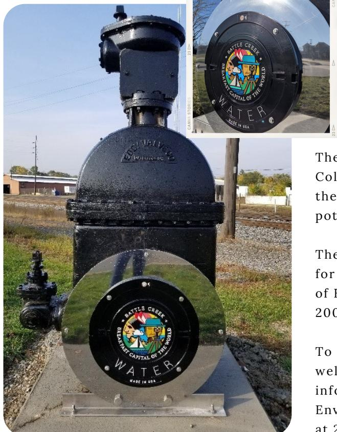
The second valve sits at the Verona Pumping Station, 250 Brigden Drive. This one is a 30-inch Darling valve, also cast in 1957. The Darling Valve Co. was in Williamsport, Pennsylvania.
