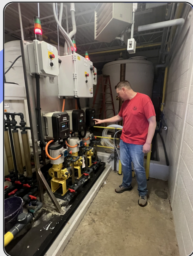
Verona teammate Josh is adjusting the sodium hypochlorite (chlorine) feed rate that is used to disinfect the drinking water and kill harmful bacteria.
